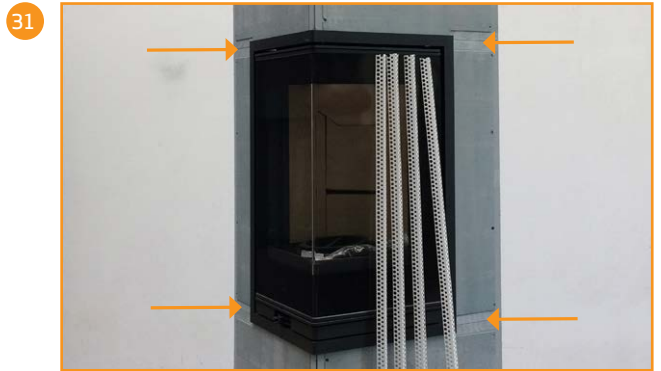
Mount self-adhesive joint tape in the filling trace. Then cut the corner strips in appropriate lengths with a large pair of scissors
