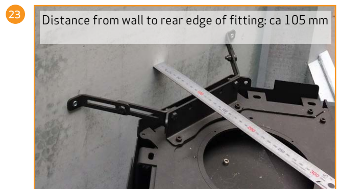
Mount the fitting for the whole rear piece
