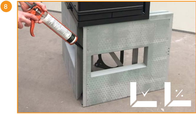
Push the front pieces together and glue them so that the bevels fit together
