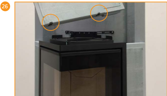
Mount the two upper front pieces with two fittings
