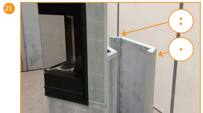
Glue the three upper rear pieces together with the side pieces and fasten with three screws
